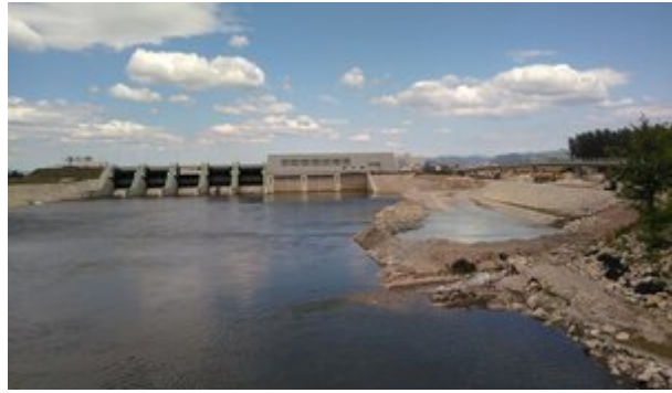
Brezice hydropower plant in Slovenia © Pippa Gallop, CEE Bankwatch Network
