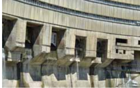
Location of reconstruction works at the Enguri dam
